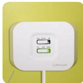
When the iT500RX Receiver and the iT500 Thermostat are paired then the light will be green.
